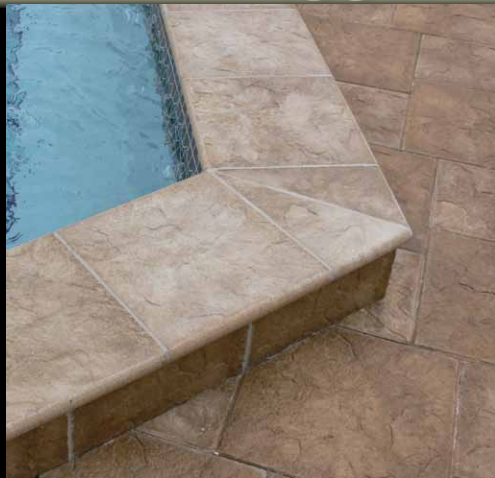
Raised pool beam and two-sided coping.
